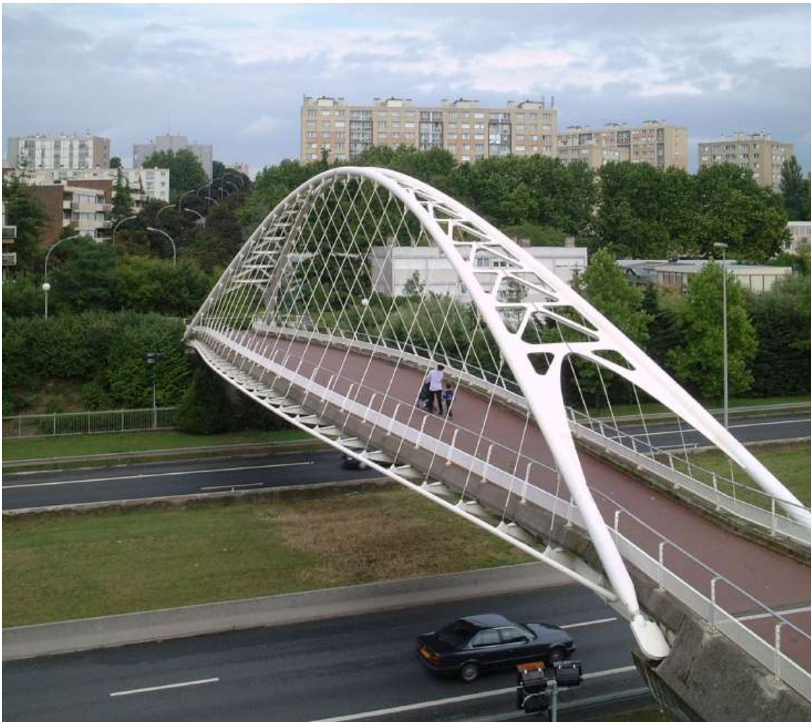
Figure 1.2.17 – A photograph of the Oudry-Mesly Footbridge [6]
