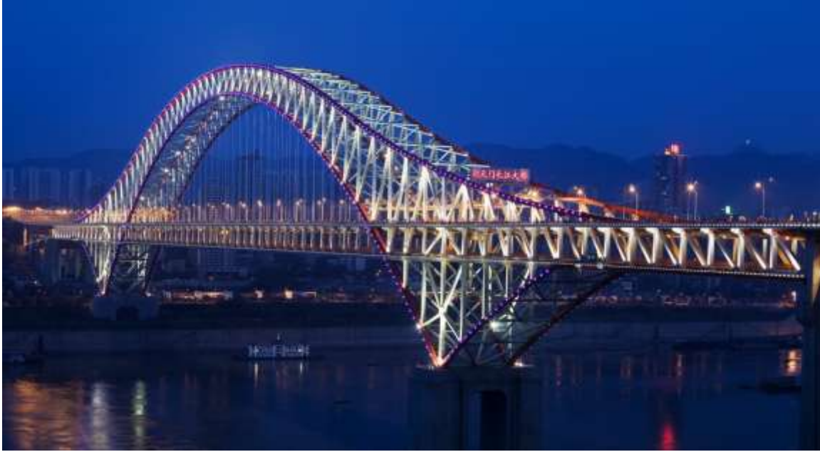
Figure 1.4.1 – The Chaotianmen Bridge [13]
