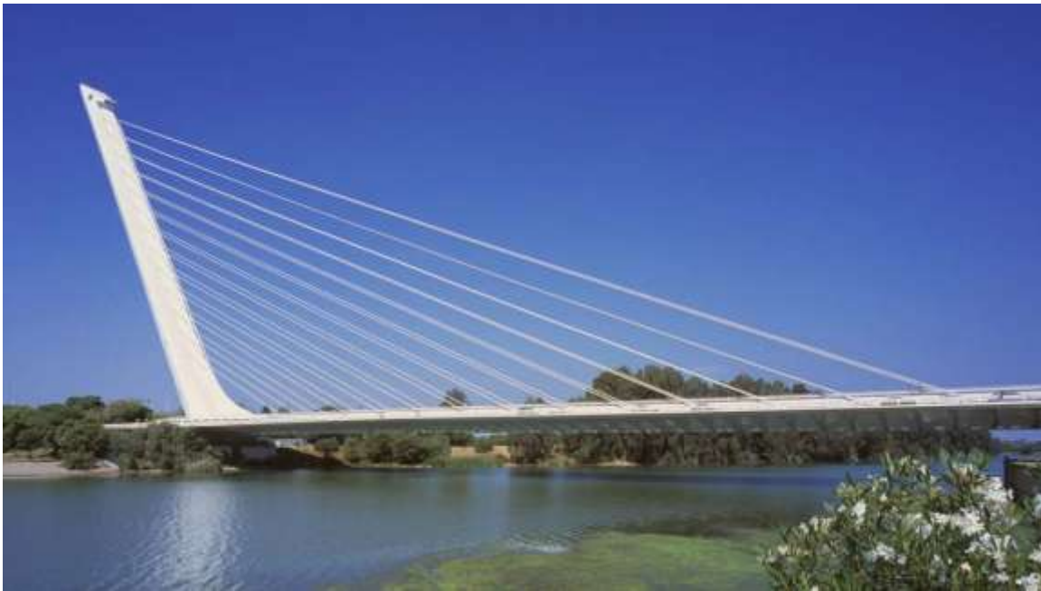
Figure 1.2.18 – A photograph of the Alamillo Bridge [7]
