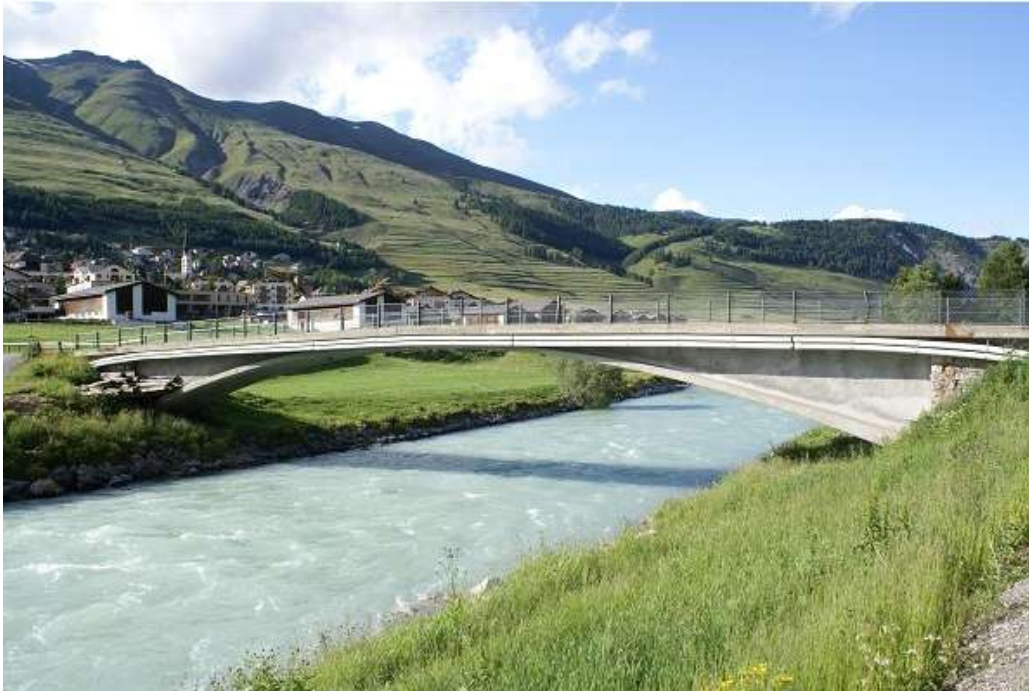
Figure 1.2.4 – A photograph of The Zuoz Bridge [2]
