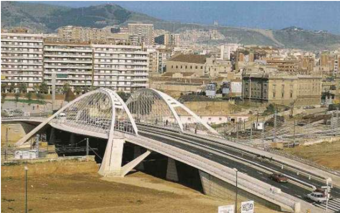
Figure 1.2.16 – A photograph of the Bach de Roda Bridge [5]
