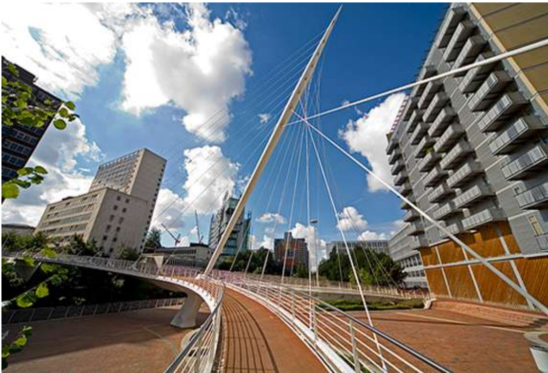
Figure 1.2.19 – A photograph of the Trinity Footbridge [8]
